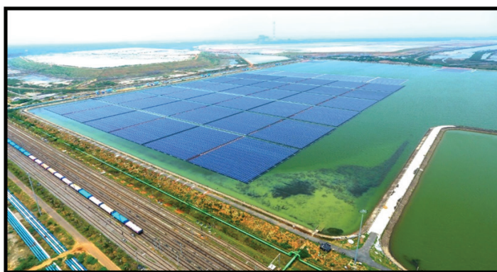
The floating Solar PV Plant at NTPC, Simhandri, commissioned by BHEL
